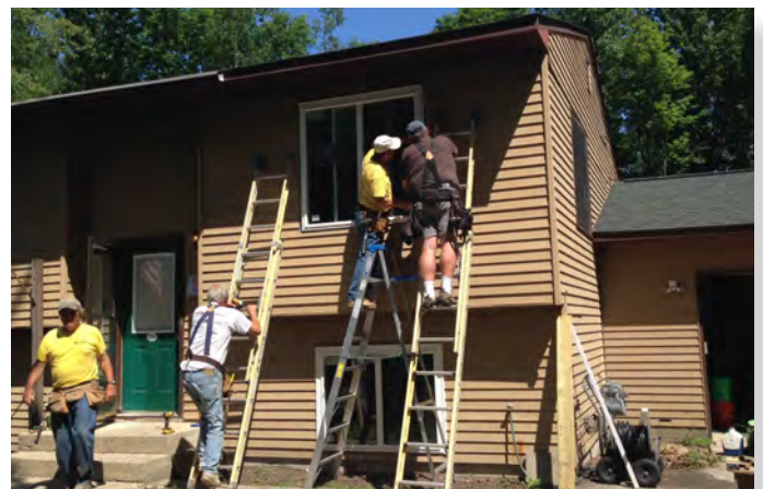
Home repair programs are critical tools to preserve and maintain existing housing.
