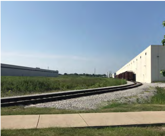
Rail access to the LogistiCenter is being expanded to serve more sites for development.
