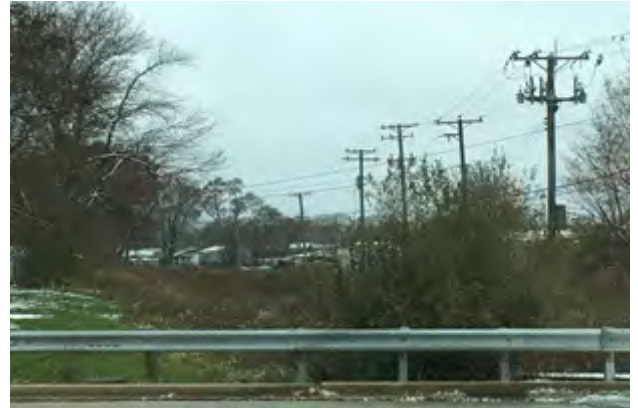
Overgrown vegetation in Lansing Ditch, west of Torrence Ave.
