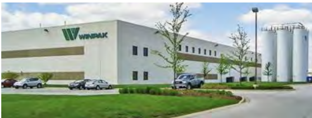
Winpak facility within the LogistiCenter.
