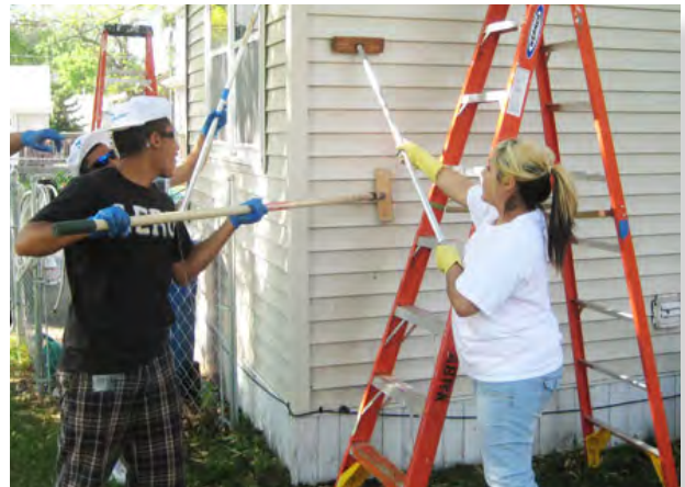
Enforcement of building codes holds property owners responsible for health and life safety.
