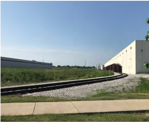
Rail access to the LogistiCenter is being expanded to serve more sites for development.
