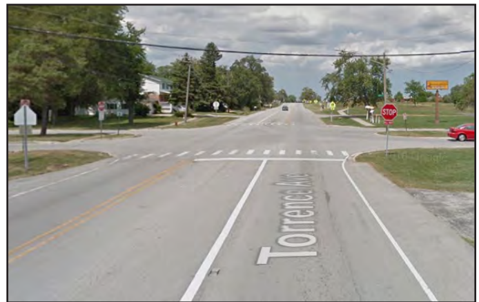
The intersection of Torrence Ave and 223rd Street, Torrence Ave is classified as a Major Collector and 223rd Street is classified as a local street.
