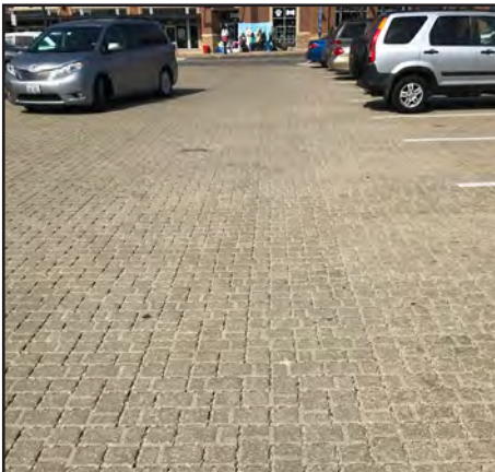
BMP1: Permeable Pavement
