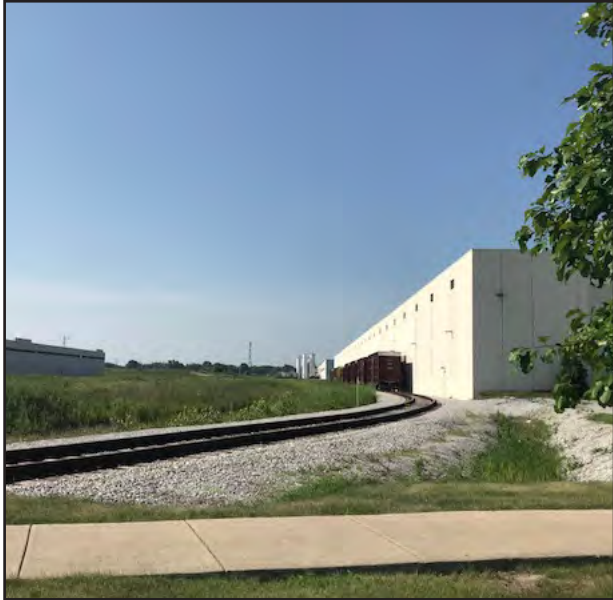
Rail spur in the LogistiCenter is an important asset to attract investment.
